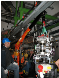
Installation of station B7R1
