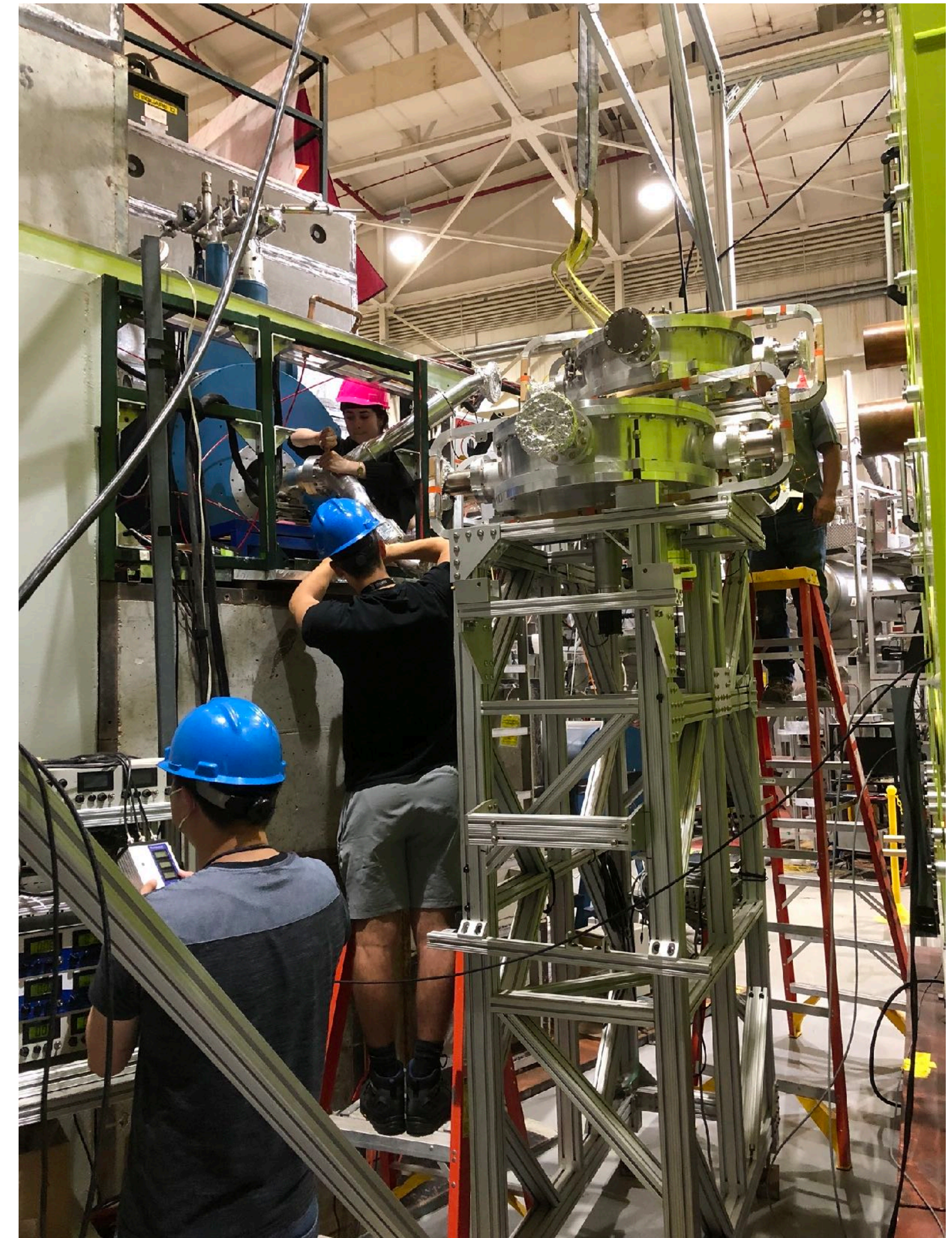
Switchers being installed
